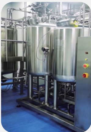
500L Dosing and Cleaning In Place (CIP) System
